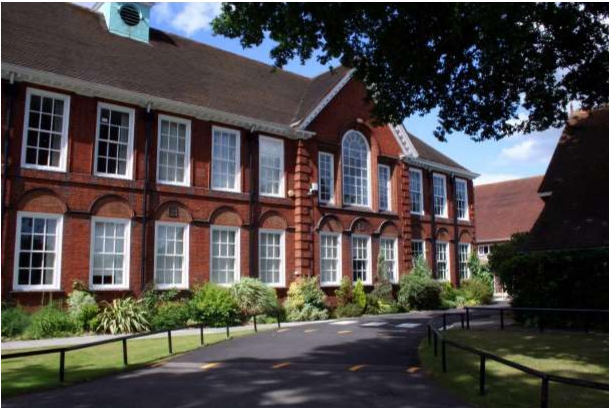
Front View of Main School Building
