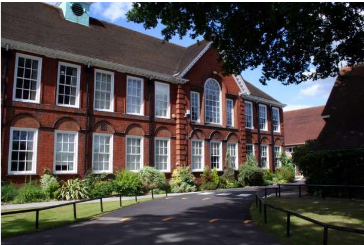
Front View of Main School Building
