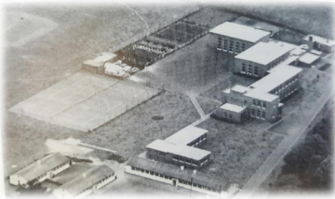
The original school buildings from 1955...
