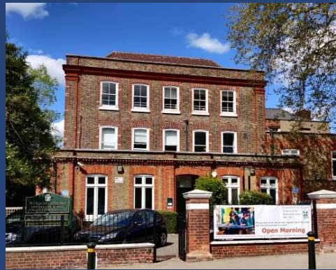
St Christopher's The Hall, Beckenham
