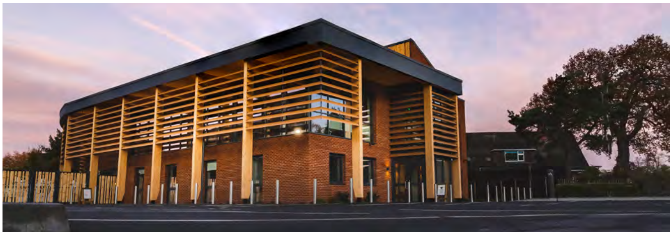
Senior School building photography by: Trevor Smith
