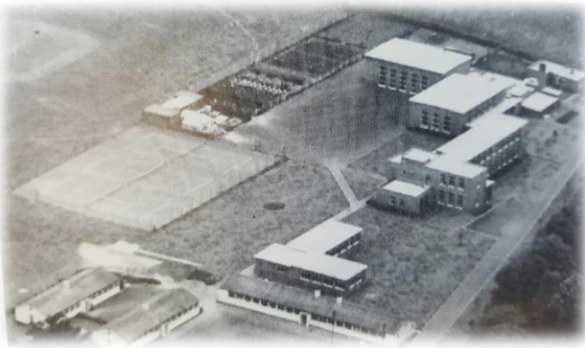
The original school buildings from 1955...
